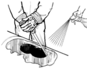
Hand Sawing Asbestos Cement Pipe
